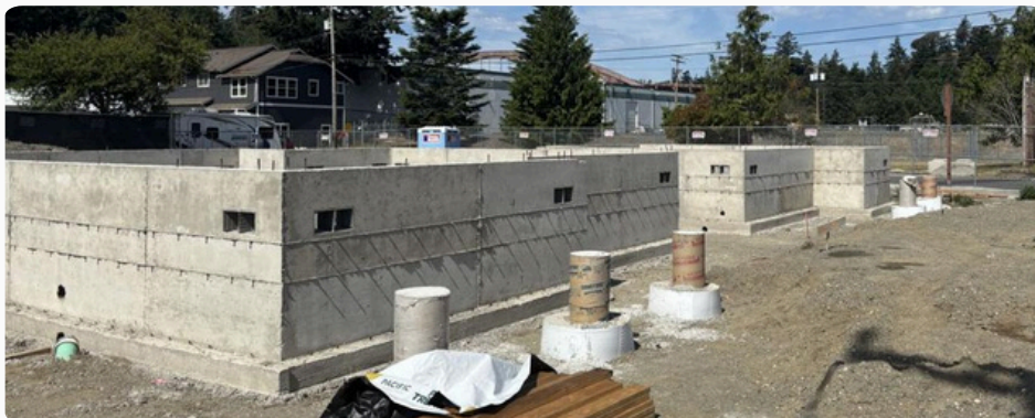
June 2026: Stem Walls Poured at Caledonia Cottages in La Conner
